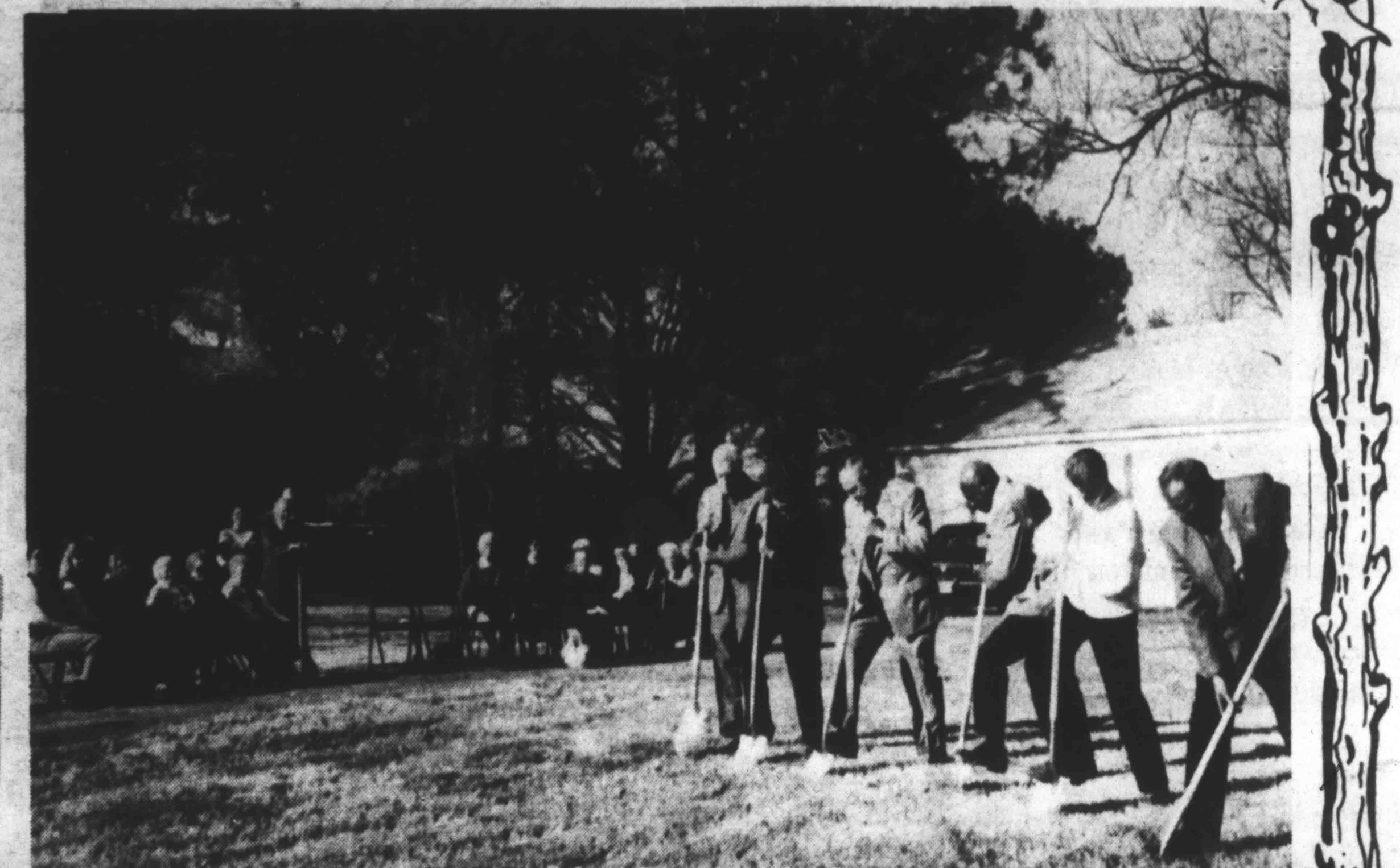
GILT-CLAD SHOVELS broke ground Friday for the new Lauderdale County Library, on the former Jack Palmer home site on Lafayette in Ripley, across the street from the Farm Bureau Building. Mrs. Palmer, who now resides in Memphis, contributed the invocation; County Executive Rozelle Criner, who presided; Susan Marvin, chief executive of Marvin Windows of Tenn., whose Ripley plant will contribute windows and doors to the project; and Bill Klutts, chairman of the Library's Board of Trustees. First to dig were, from right, Ripley Mayor Richard Douglas; Tim Duke, representing the architects, William Haizlip + Pounders, of Memphis; The Rev. Robert Flagg, of Henning, a County Commissioner who brought the invocation; County Executive Rozelle Criner, who presided; Susan Marvin, chief executive of Marvin Windows of Tenn., whose Ripley plant will contribute windows and doors to the project; and Bill Klutts, chairman of the Library's Board of Trustees. Joe Graves provided the shovels, on behalf of McA-doo Builder Contractor, of Union City, which won the construction contract on a low bid of $412,000. Completion of the new building is expected in July.
